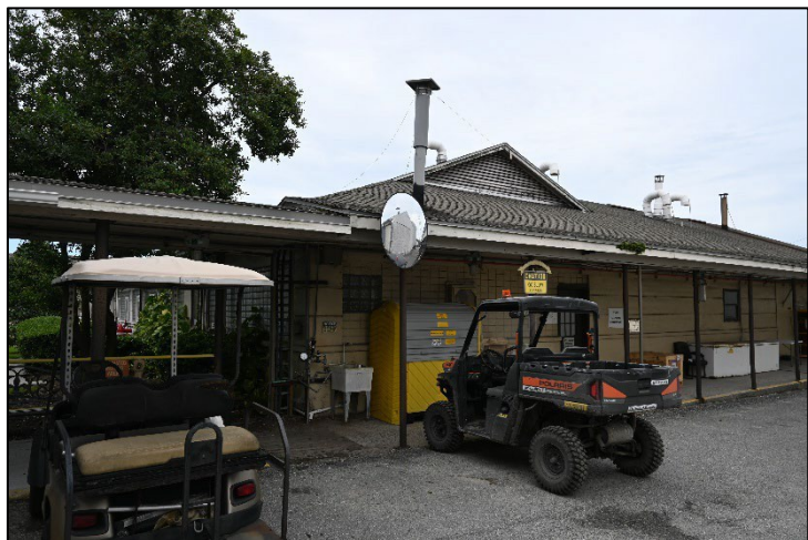
Figure 3. Office building, facing east.
